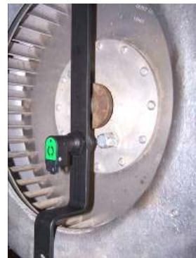
CRARY FAN SENSOR INSTALLATION
