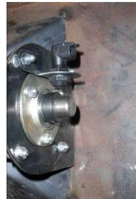
AUGER SENSOR INSTALLATION
